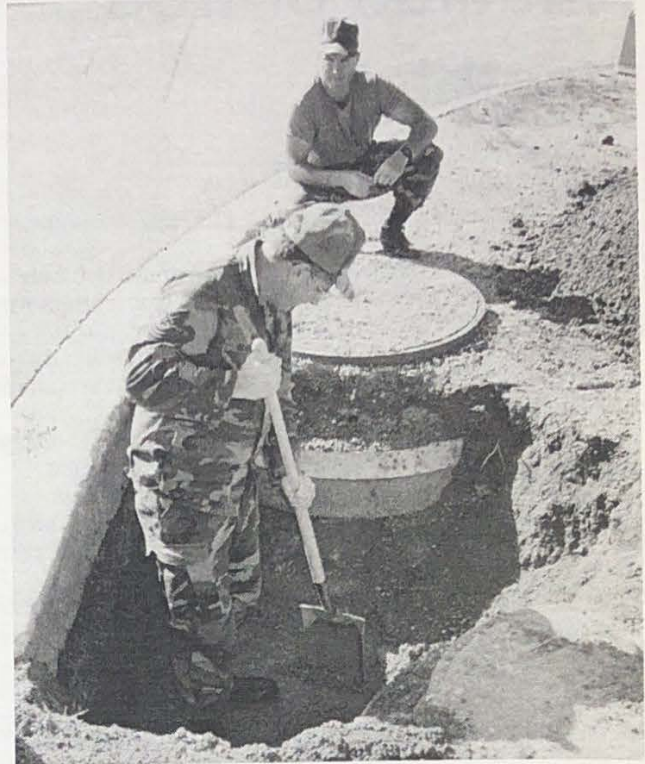
MSgt. Steven Blansett, foreground, and SSgt. Tim Givens, 507th Civil Engineer Squadron, prepare a manhole for installation of a communications conduit during the unit's annual tour at the Air Force Academy. (Photo by MSgt. Tommy Clapper)
